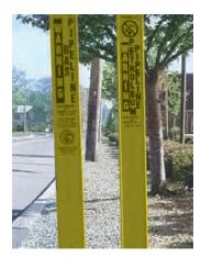
The markers display the material transported in the pipeline, the name of the pipeline operator and a telephone number where the pipeline operator can be reached in the event of an emergency.
